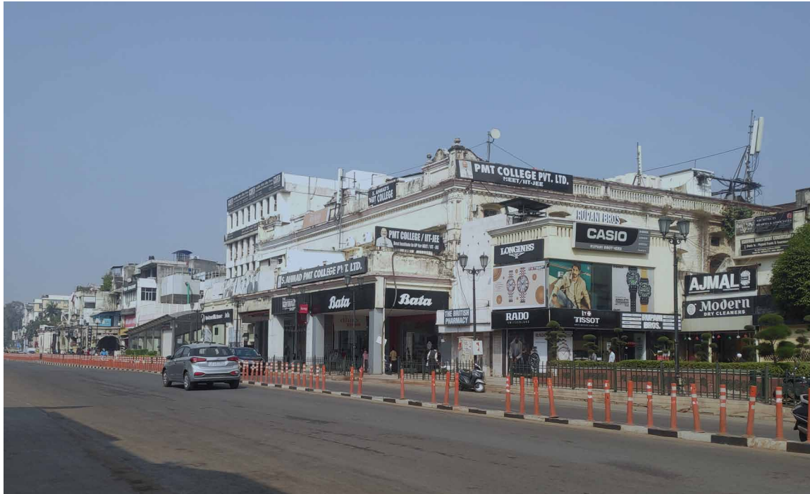
Figure 1. The view of the heritage street Hazratganj (Source: The authors)
